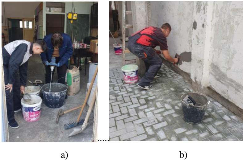
Figure2 – Practical activities at LTCPM Arad: a) mortar mixing, b) plastering.
