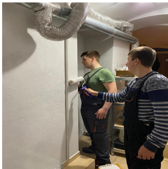
Finishing and painting works at Homefix, Wrocław
